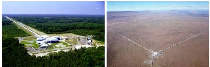
Aerial view of the LIGO gravitational-wave detectors, situated in Livingston Louisiana (upper panel) and Hanford Washington (lower panel). Each instrument is a giant Michelson laser interferometer with arms 2.5 miles long.
